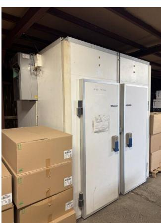
A large white industrial unit, identified as a positive cold group (groupe froid positif), standing in a warehouse. It has two doors and is surrounded by cardboard boxes.        |
