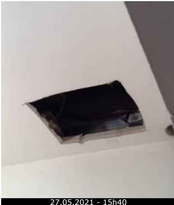
Photo 23 (WC / Plafond / Trou(s))
